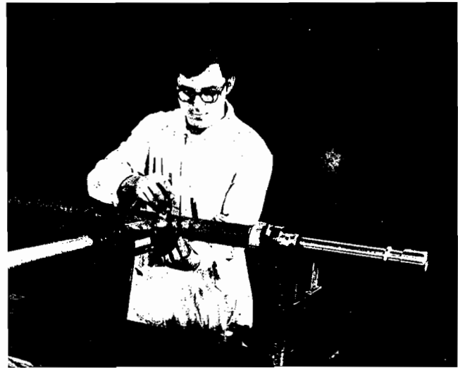
Figure 3. D-Gun Coated Piston Rod.
